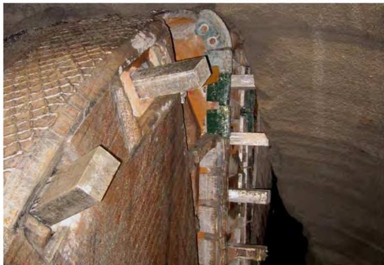
Figure 10 – Heavy block rippers, BWARI Project, Columbus, Ohio [13]
